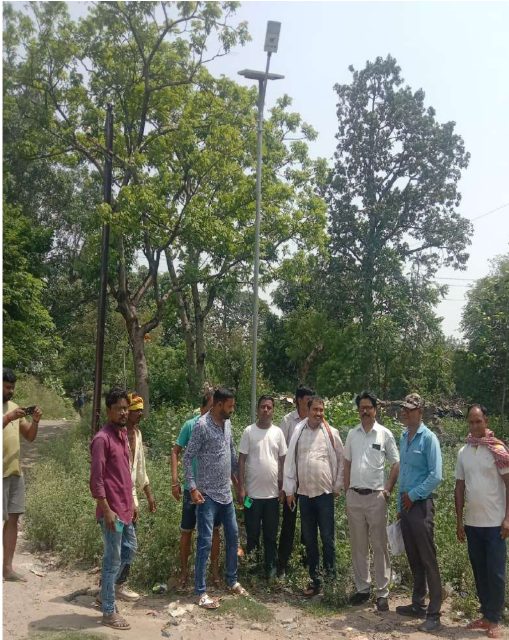
Solar Street light installation at Argada on 02/06/2025
