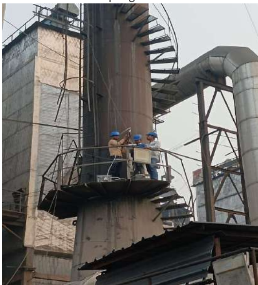
Sampling taking from stack
